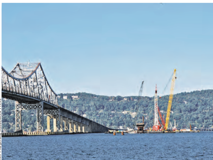
The Tappan Zee on Sept. 27, with cranes for preconstruction work
